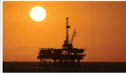
Oil and gas pipelines Offshore platforms
